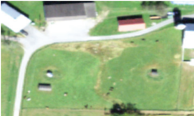
Stormwater Erosion Feature Before (2019 aerial)
