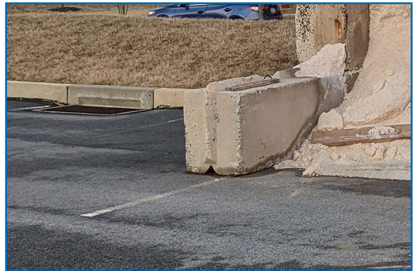
Rock Salt Storage and Storm Drain
